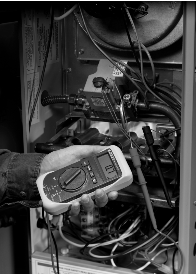
Figure 19. Fluke 16 in the microamps mode testing the flame rectification circuit.
